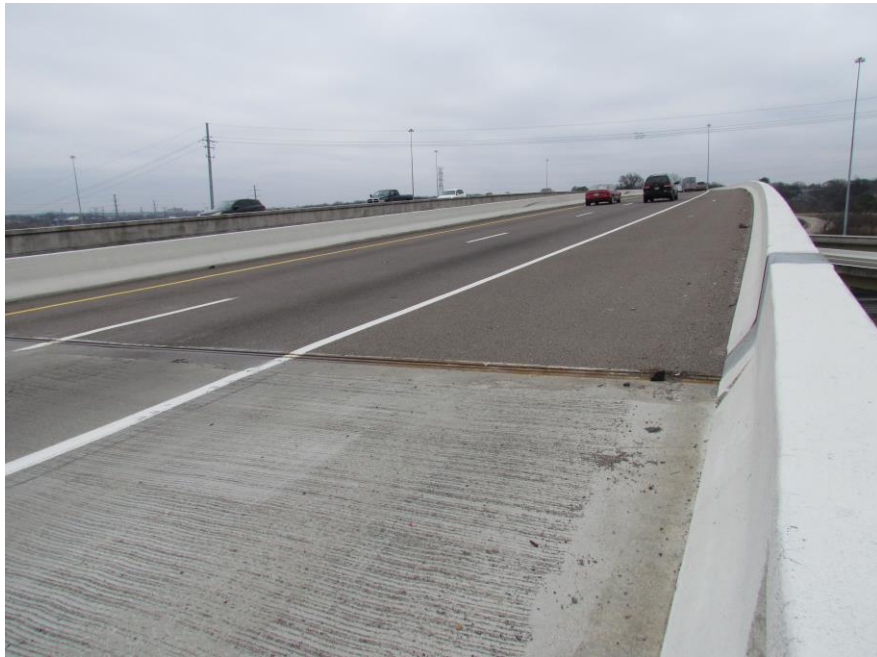
VIEW ACROSS TOP OF WEARING SURFACE I440
