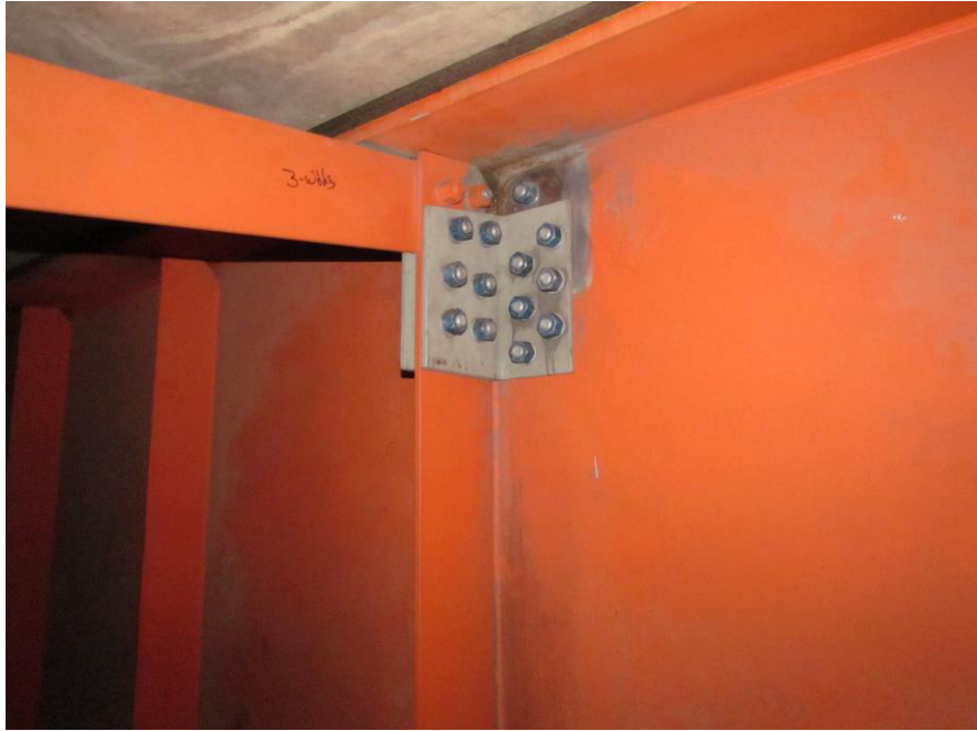
TUB "B" REPAIRS CLOSE-UP - TYP.
