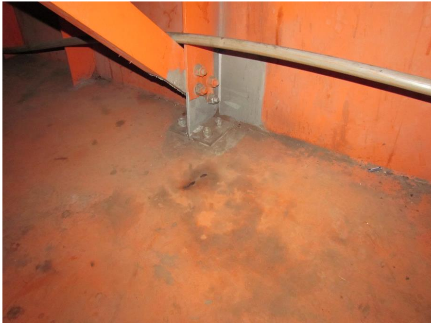
TUB "B" REPAIRS CLOSE-UP - TYP.
