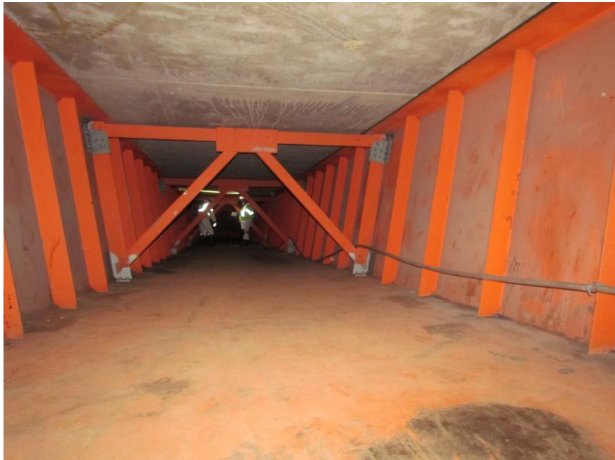
TUB "B" DIAPHRAGM #1 SP. #1 REPAIRS TYP
