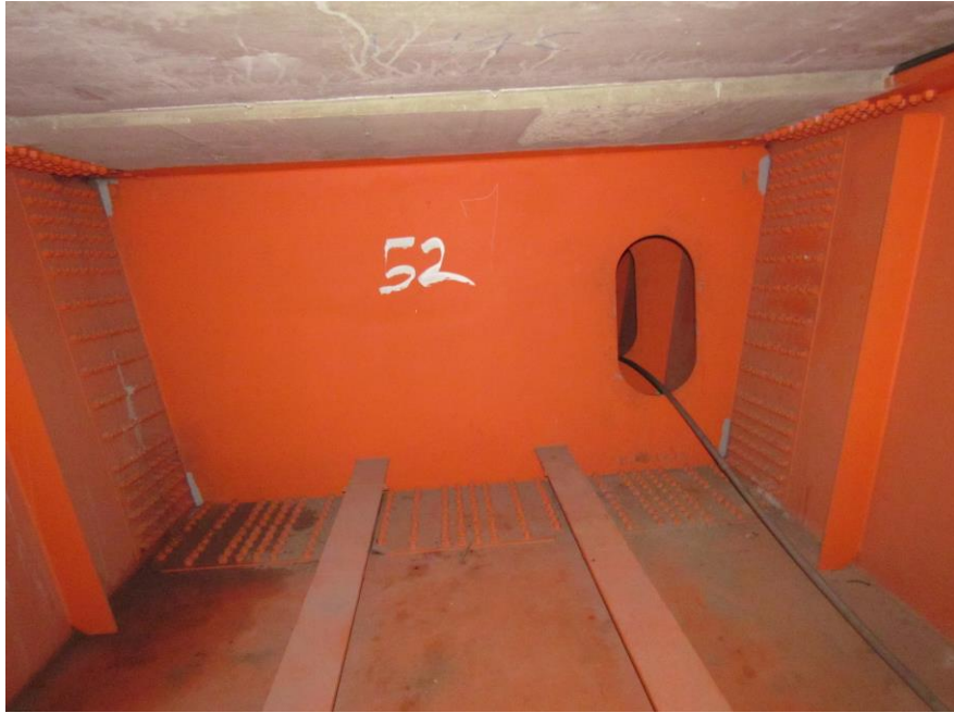
END VIEW AT SPAN #1
