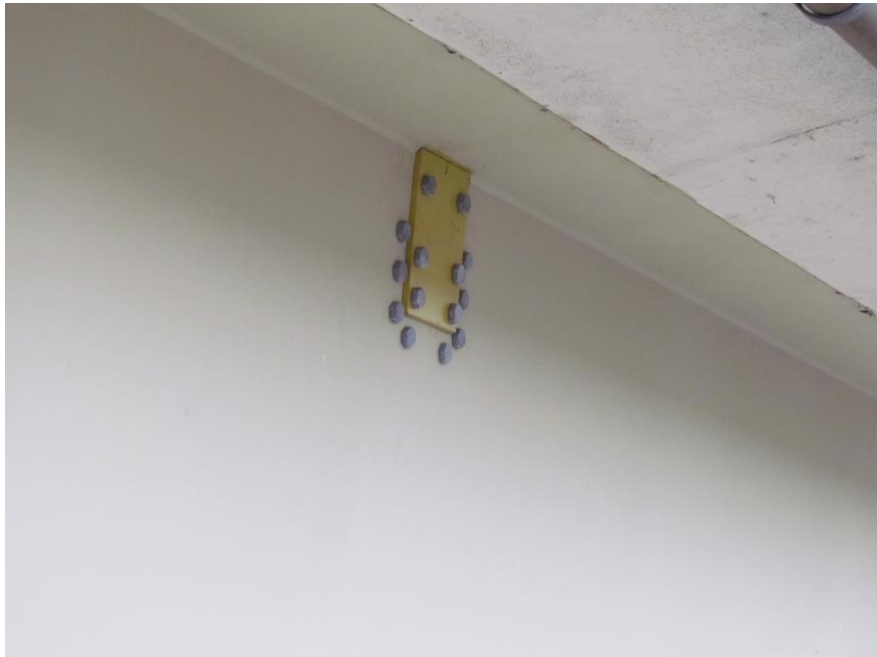
TUB "B" CLOSE-UP VIEW REPAIR PLATE OUTSIDE
