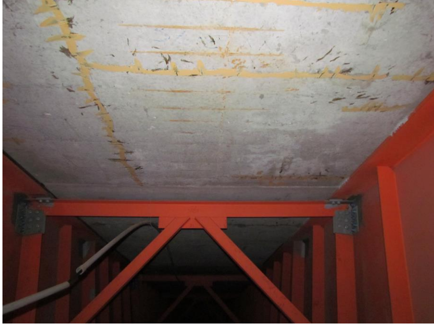
TUB "B" DECK PANELS SP. #3 W/ REPAIRS
