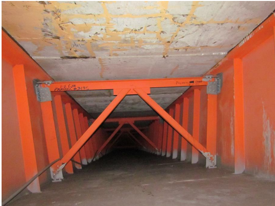
TUB "B" DECK PANELS SP. #3 W/ REPAIRS
