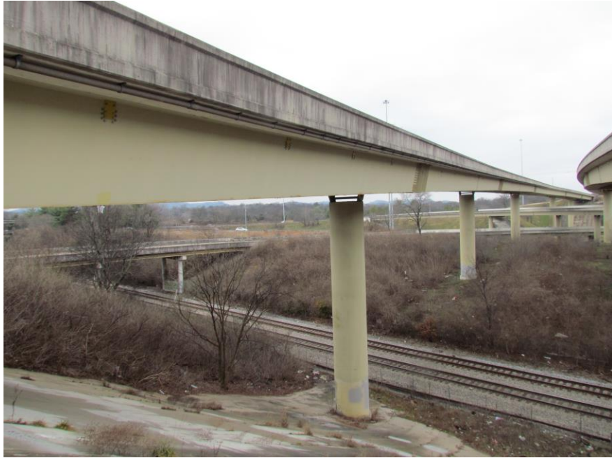
CLEARANCE VIEW LT. SIDE
